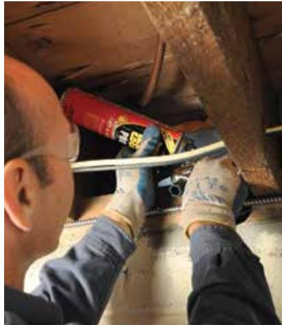
Use low-expanding foam when sealing board insulation against wood rim joints.
