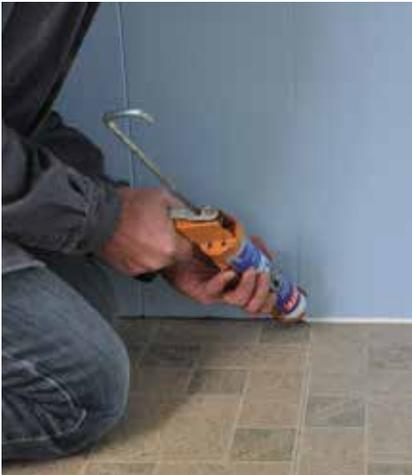
When caulking, hold the gun at a slight angle, and work backward along the seam rather than pushing forward.
